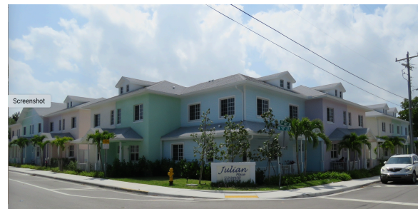
Exterior view of Julian Place
