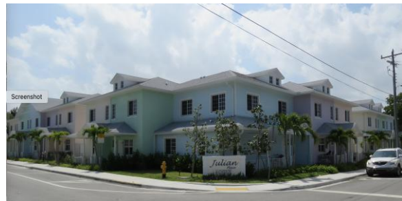
Exterior view of Julian Place
