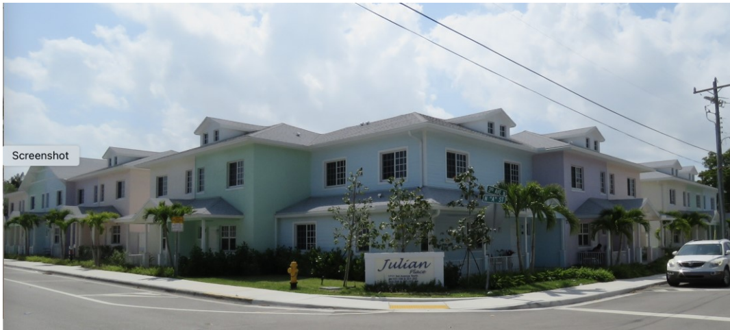
Exterior view of Julian Place
